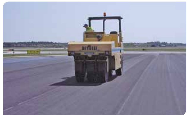
Compaction is often specified for airport jobs
