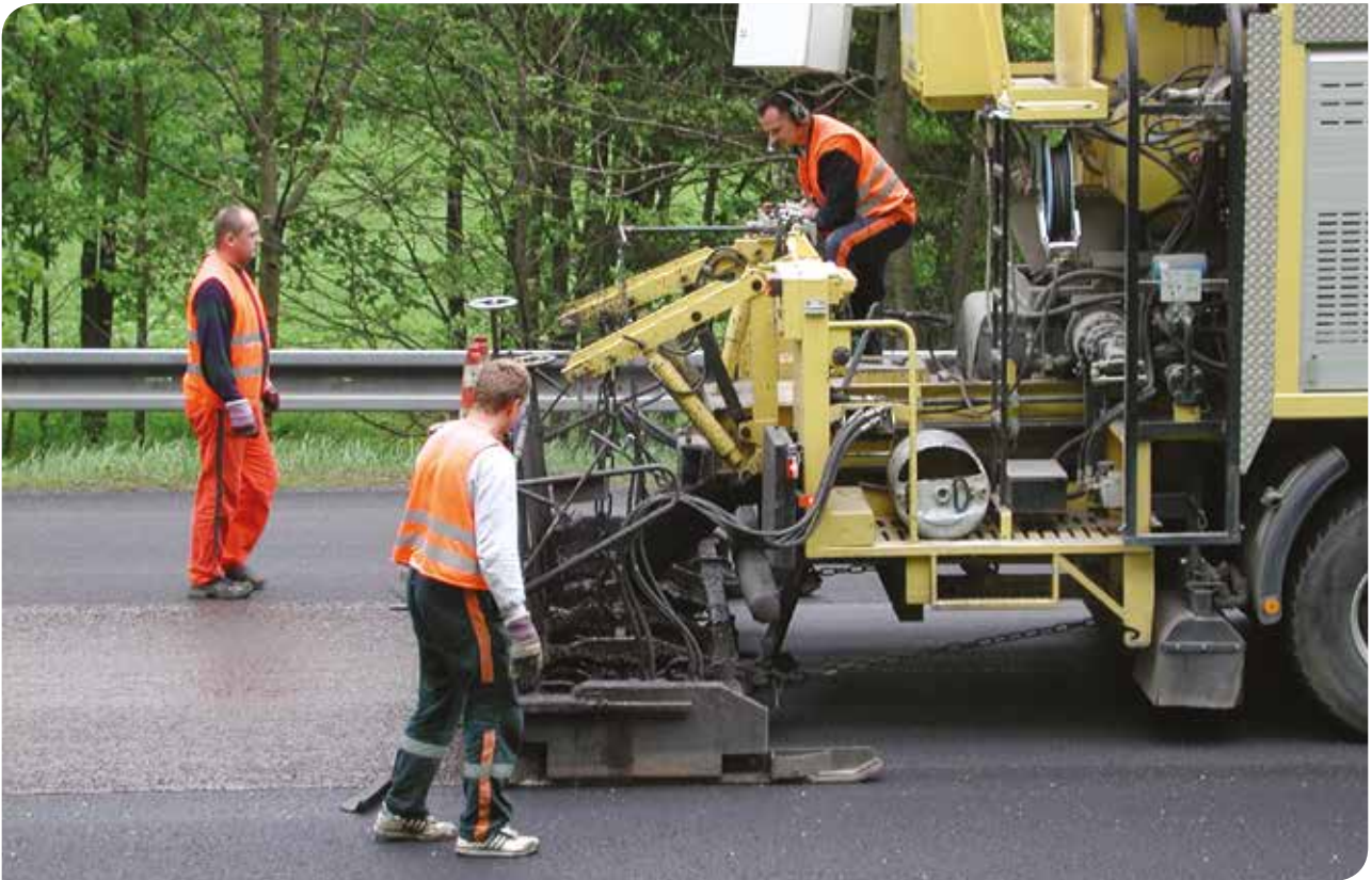
Microsurfacing in Czech Republic with Redipave phosphoric acid system
