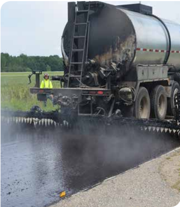
As observed, all spray nozzles were properly aligned and not clogged.
