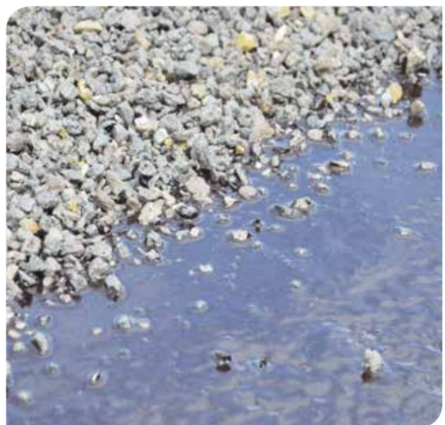
The aggregate appeared to have proper embedment into the emulsion between 50% to 70% of its width.
