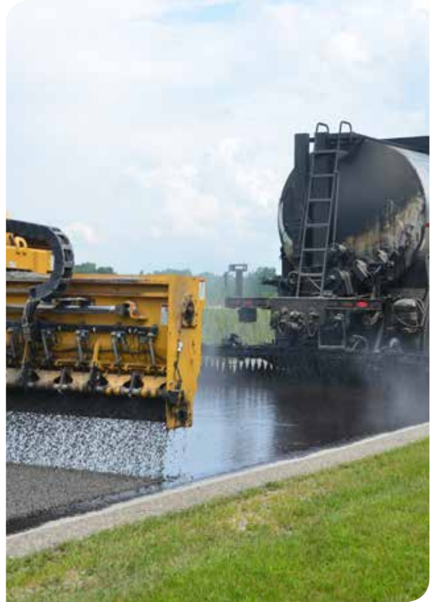
The aggregate appeared to have proper embedment into the emulsion between 50% to 70% of its width.
