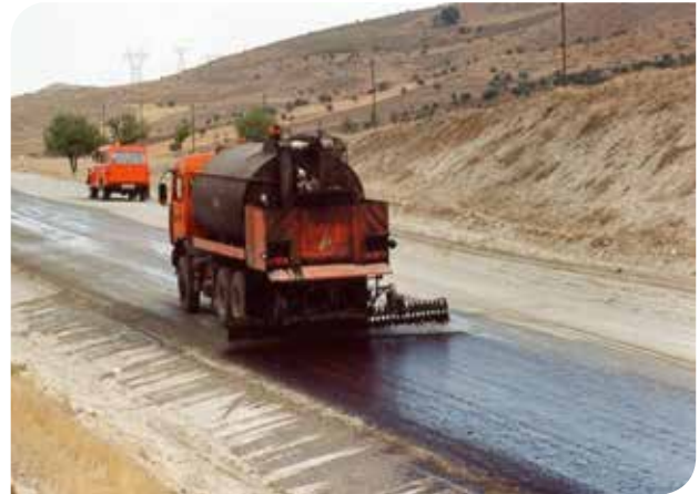
Prime coat application with asphalt emulsion
