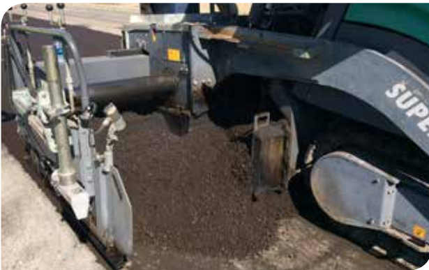
Cold in-place recycling – Courtesy of Pavement Recycling Systems (PRS)
