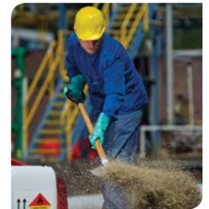
Use vermiculite or perlite to clean up small spillages
