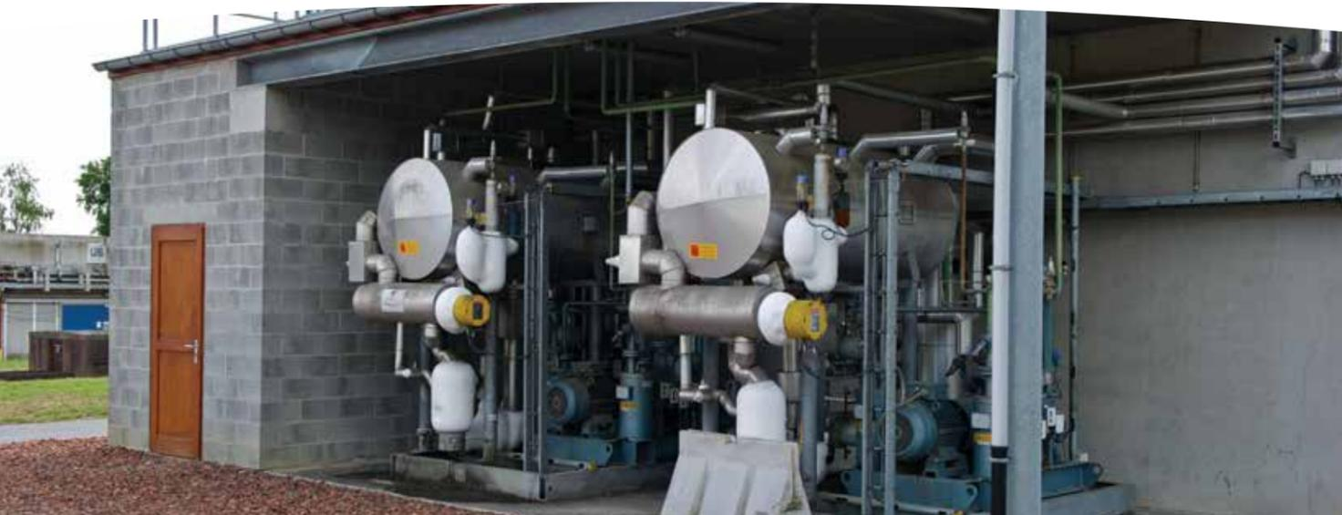
Two cooling units, alternately operating, fully independent of each other
