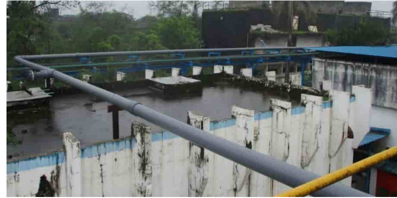
Connected Pipeline to transfer rainwater to storage tank.
