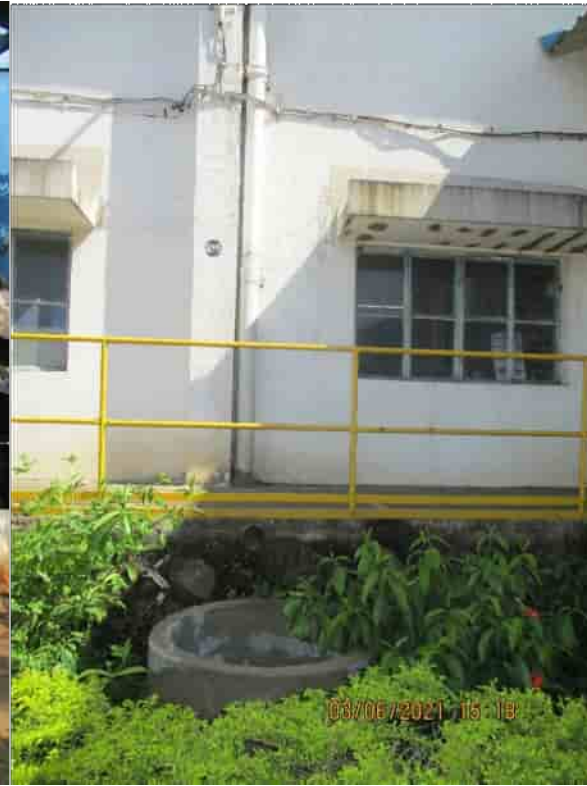
2. Rainwater recharge pit of Building roof
