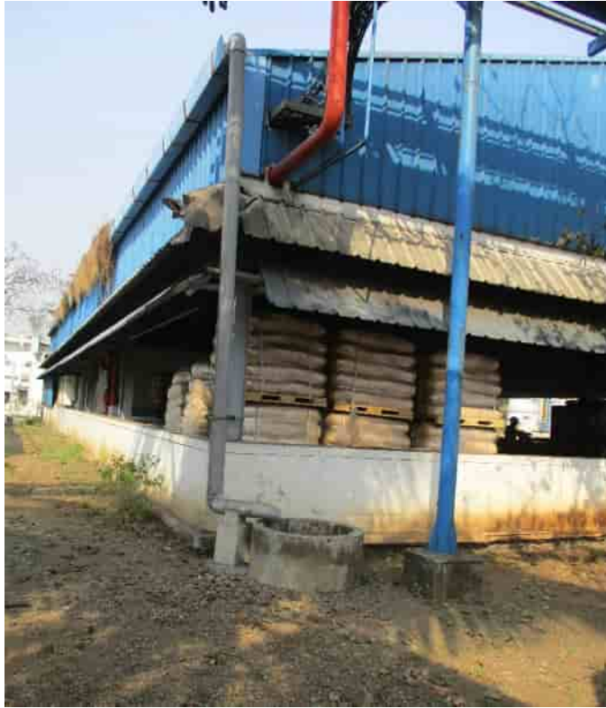
1. Rainwater recharge pit of Warehouse roof
