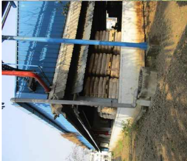
1. Rainwater recharge pit of Warehouse roof
