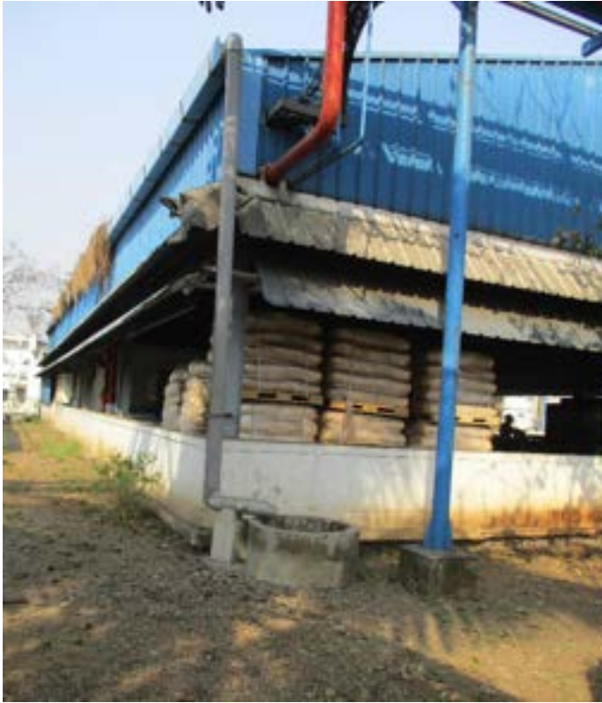
1. Rainwater recharge pit of Warehouse roof
