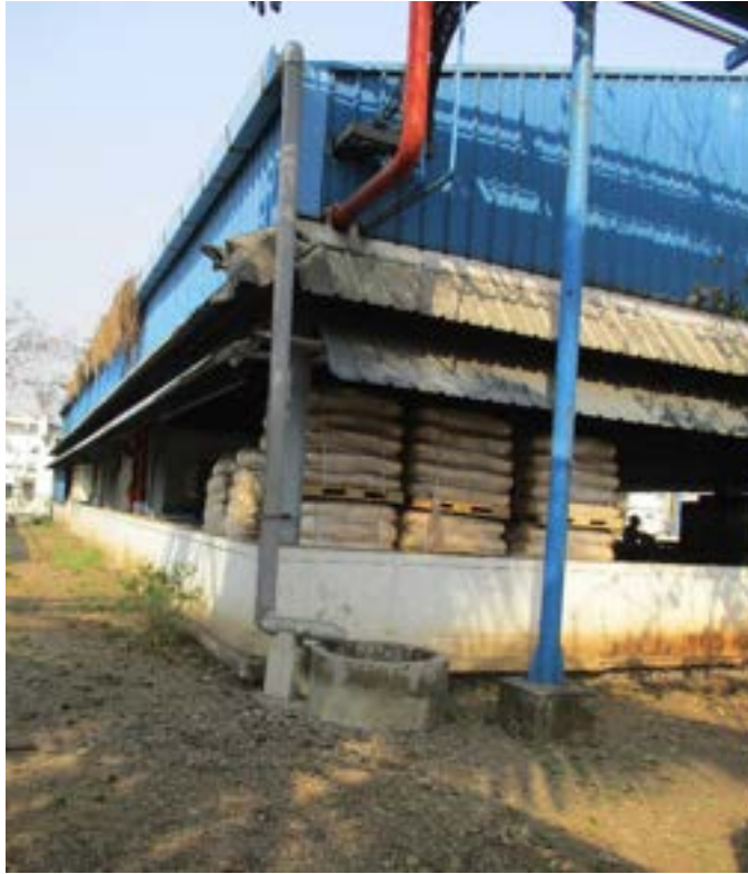
1. Rainwater recharge pit of Warehouse roof
