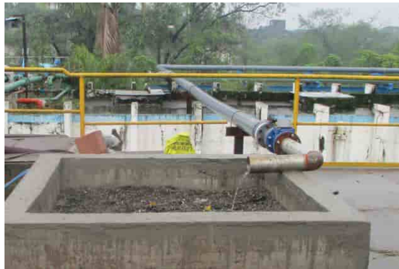
Roof top rainwater collection
