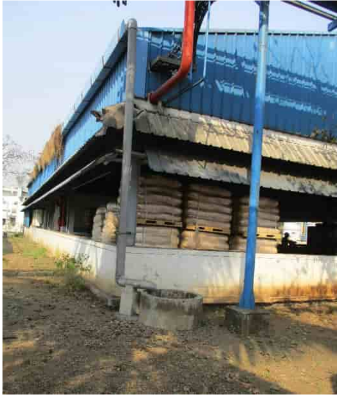
1. Rainwater recharge pit of Warehouse roof
