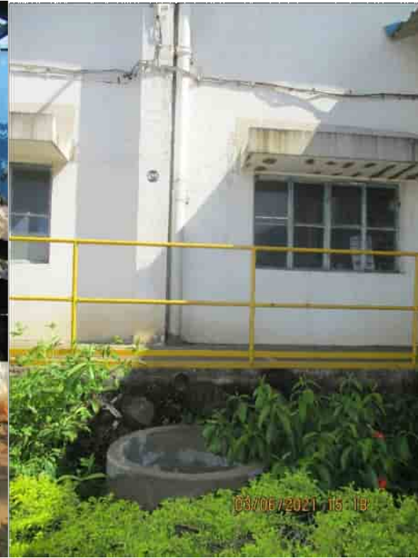
2. Rainwater recharge pit of Building roof
